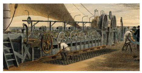
Figure 3: Part of the cable paying-out equipment on board the Great Eastern.
